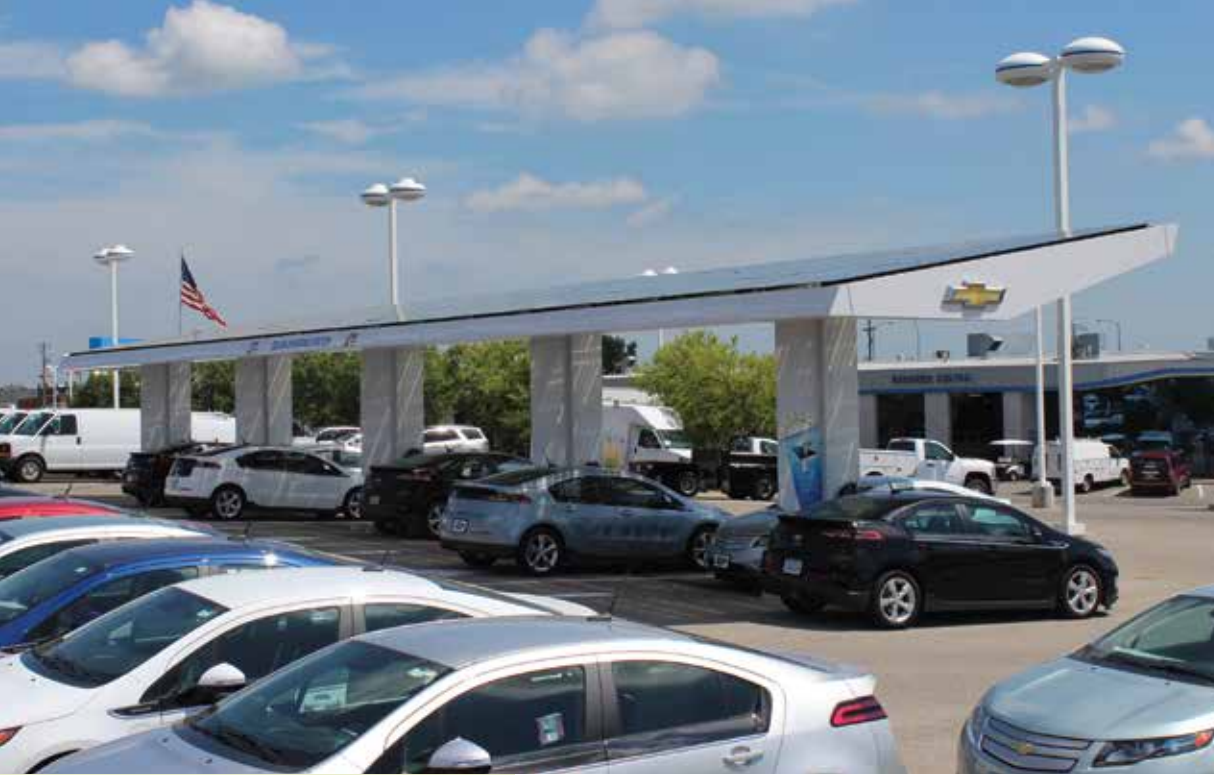
Karl Chevrolet in Ankeny has installed a solar canopy over an electric vehicle charging station.
