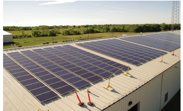
▲ Access Energy Cooperative in Mt. Pleasant installed 100 kW of solar panels on the roof of its headquarters.
