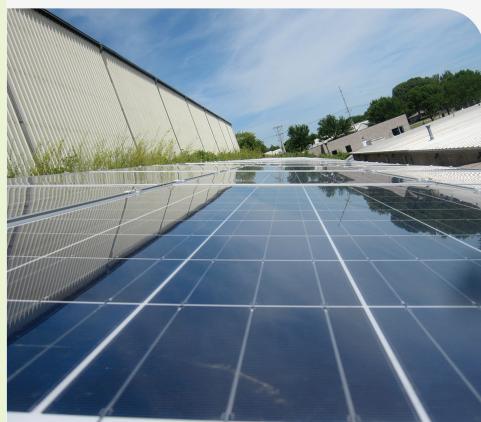
Solar and wind energy are gaining rapid momentum in the Hawkeye State.
