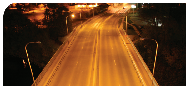
ABOVE: High pressure sodium streetlights.
