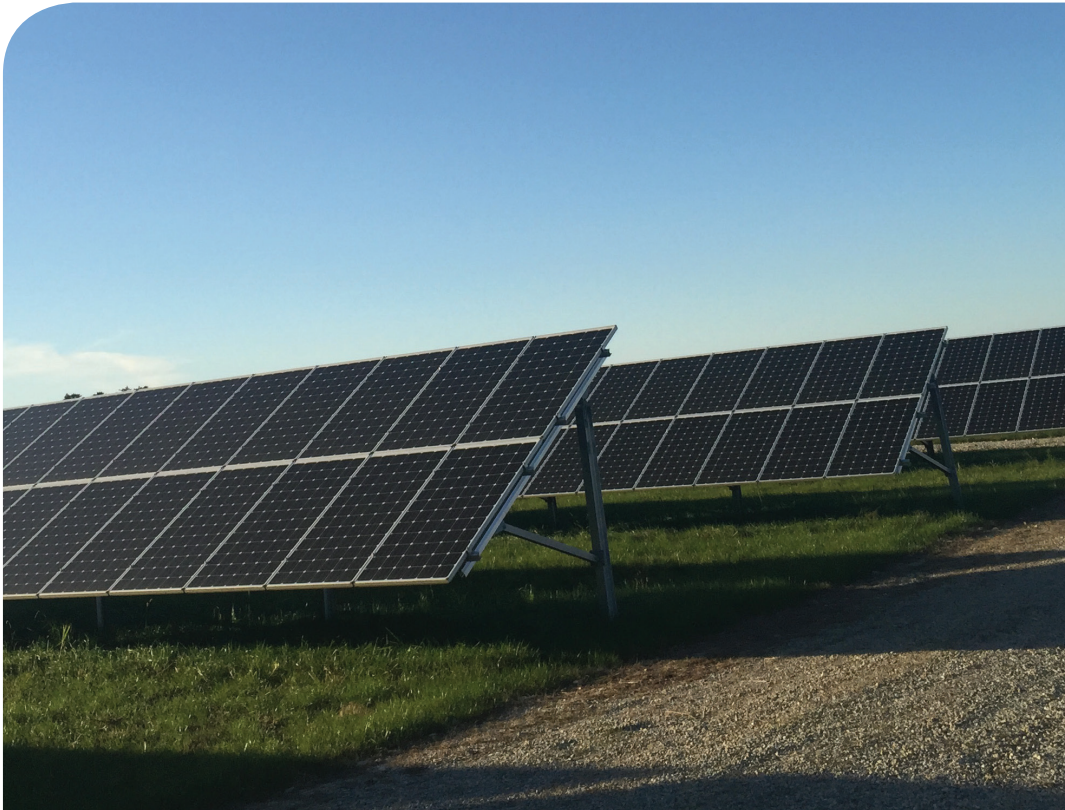
The Heartland Power Community Solar Project located on 4.5 acres east of St. Ansgar, Iowa will produce 1.2 million kilowatt hours annually once completed, enough to power approximately 125 homes.
