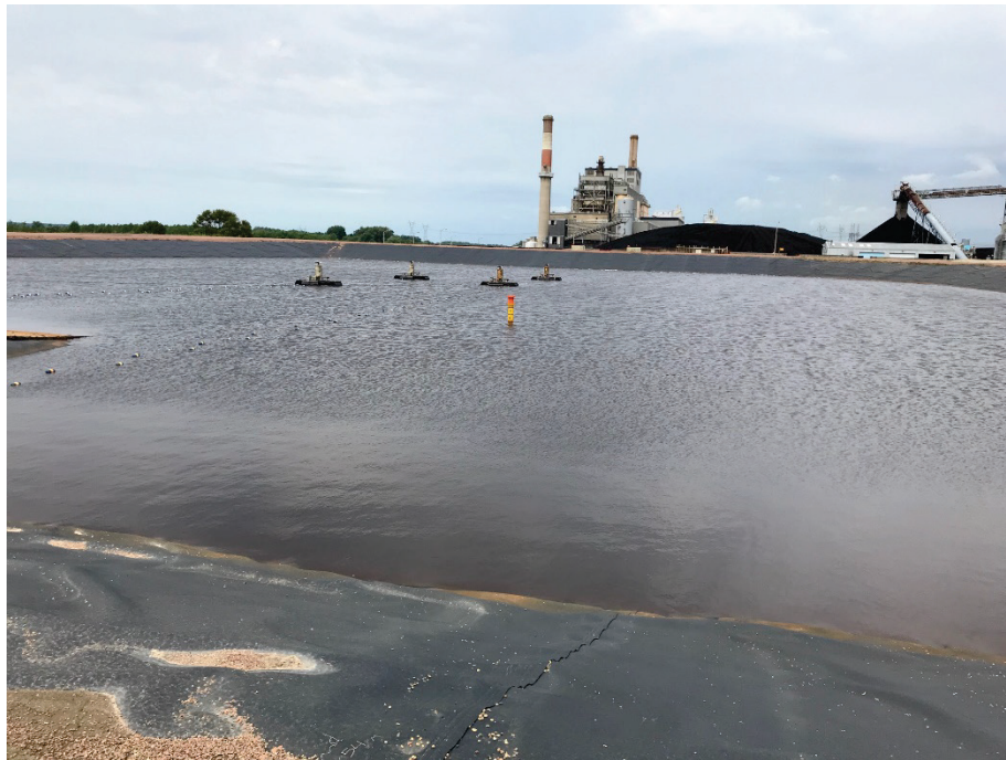
Photo 4 - 7/31/19 – Leachate pond with four evaporators deployed. Evaporators are not operating in the photograph, likely due to wind conditions.
