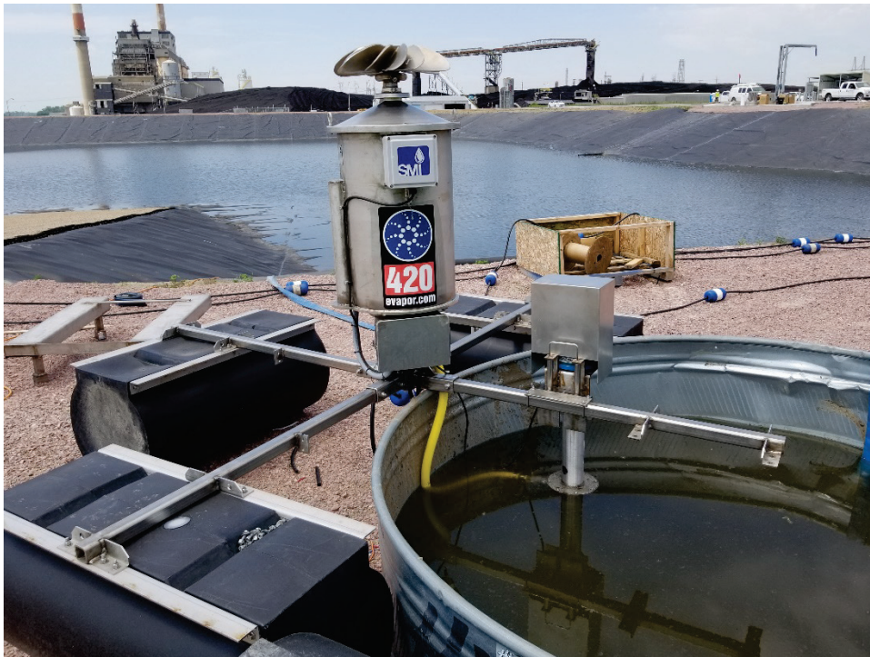
Photo 1 - 6/6/2018 – Evaporator at proveout testing with clean water. Two evaporators were deployed in April 2019. (Two additional evaporators were added July 24, 2019).
