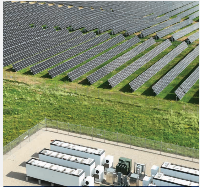
The Cedar Rapids Community Solar Garden at Deer Run, also called Alliant Energy Deer Run, is located in Linn County, Iowa. The 4.5 MW installation features a 5 MW battery energy storage system, also pictured.
