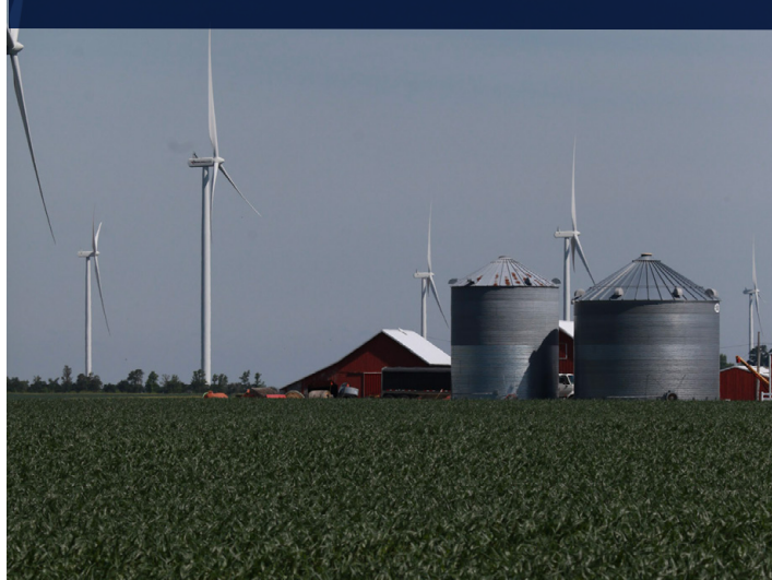
Poweshiek County Wind Farm, near I-80 in Malcolm, Iowa.
